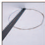
Cut hole in ceiling using template supplied.
