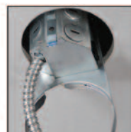
Insert plaster frame into ceiling opening.
