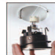
Insert trim to complete installation.
