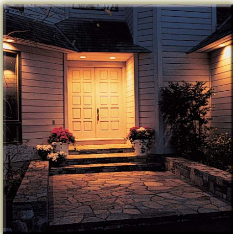
Smart Box controls 500 watts of front door lighting. (Hint: Look on the wall to the left of the door.)
